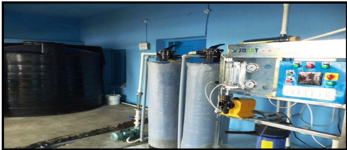
RO Water Plant Provided in Srinagar village
