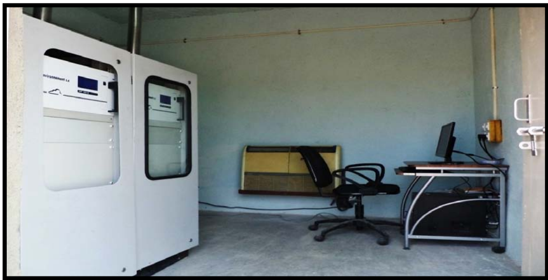
CAAQMS Station-3 installed at Mines area
